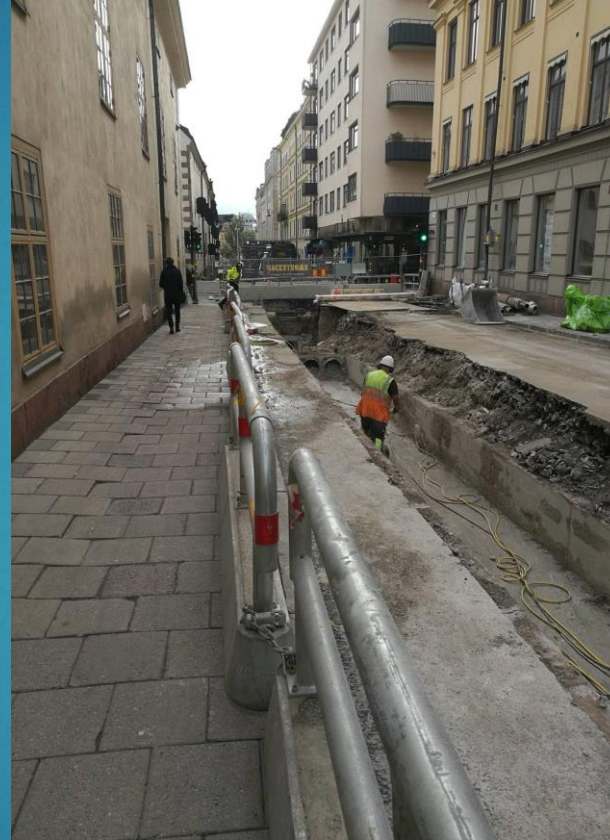
Reinvestment of district heating pipe network
