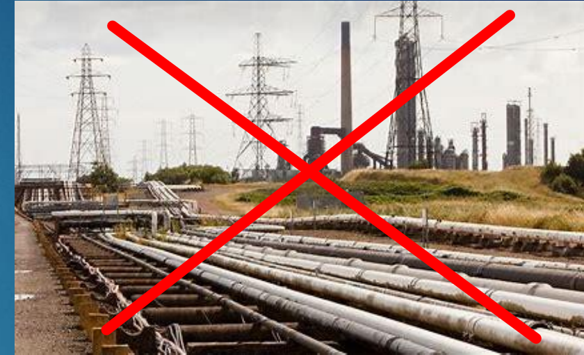
Natural gas pipe lines
