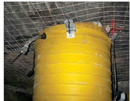
Pumped full and pressurized.
