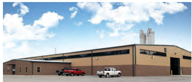
J-PAK plant in Marion, IL.
