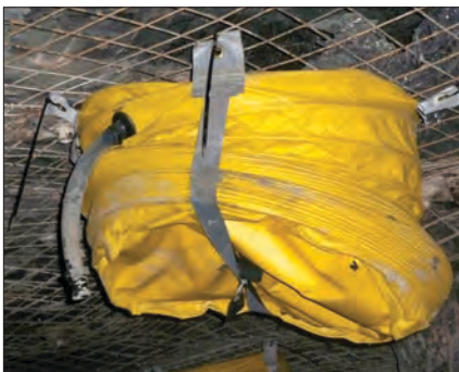
J-CRIB bag attached to wire mesh.
