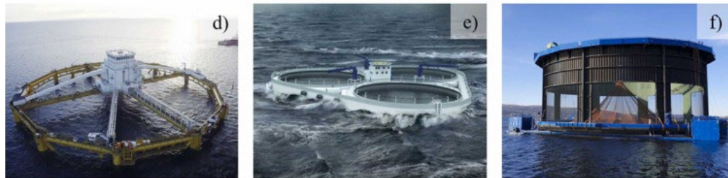
d) semi-sub "Ocean Farm" e) rigid floater "Øymerd" f) partly closed farm "Aquatraz"
