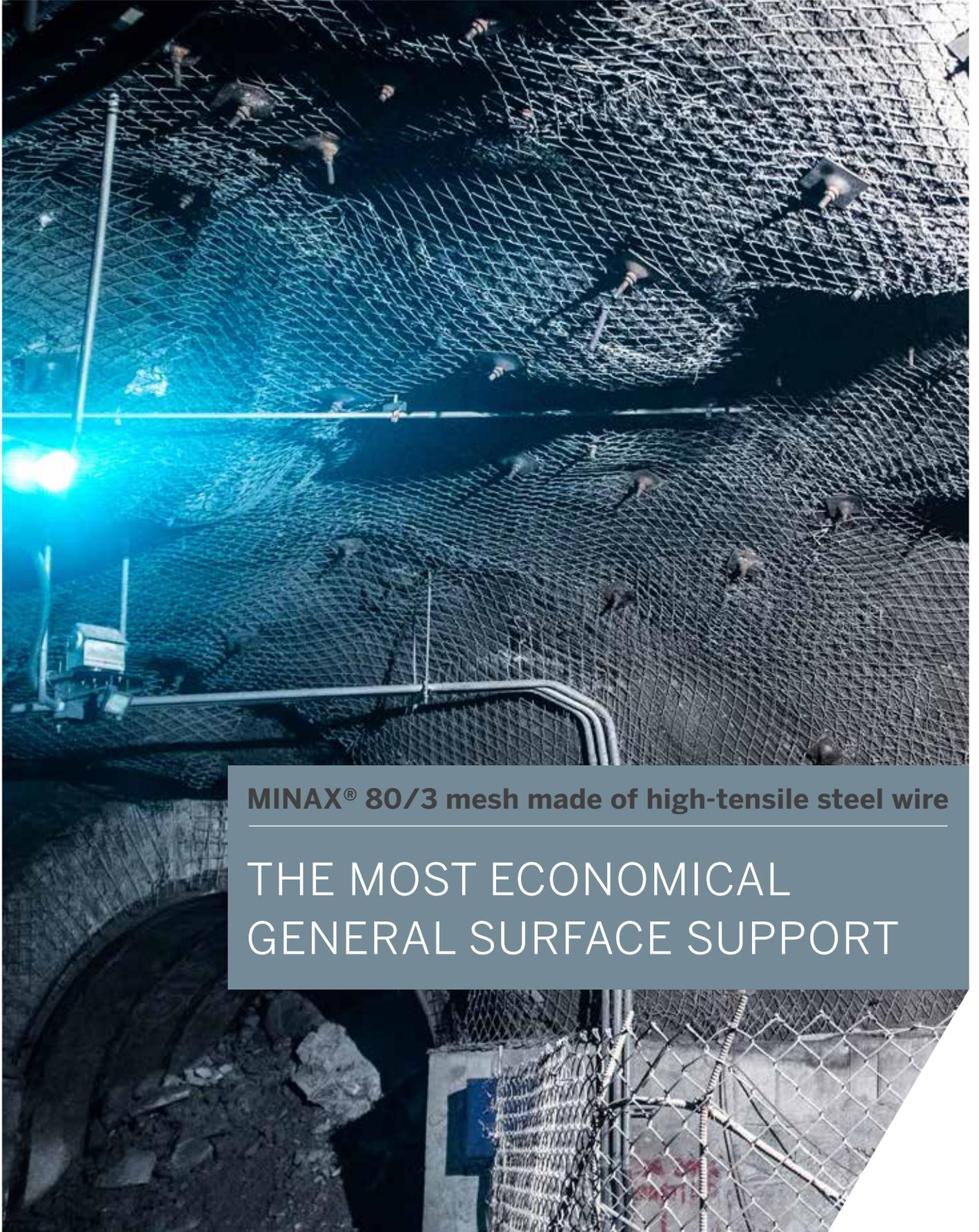
**MINAX® 80/3 mesh made of high-tensile steel wire**
